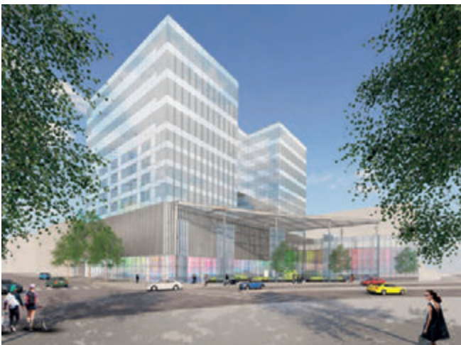
Front view rendering of the Union Tower West building showing ground floor retail space, parking on levels 2 - 4, Hotel Indigo on levels 5 - 8, and office on levels 9 - 12.
