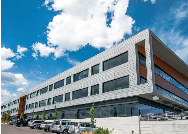
Douglass Colony Group completed the entire skin of the building as well as the roof.
