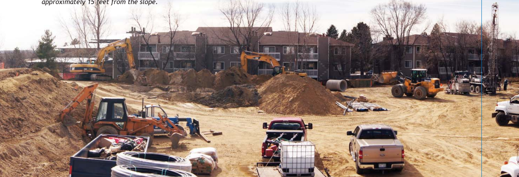
Construction was in process on the geothermal installation at Kestrel and the delegates watched as geothermal wells were being drilled 400 feet underground. ▶
