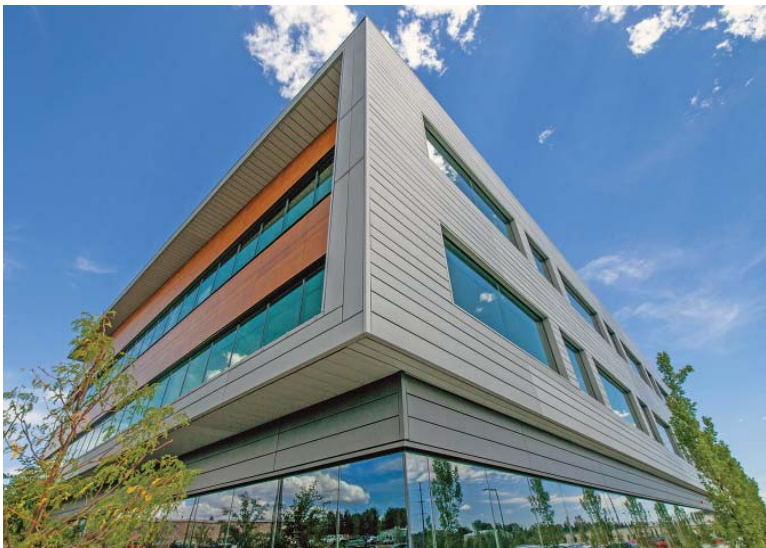
A combination of unique materials: Parklex Real Wood Panels and pre-weathered Jarden Zinc.
