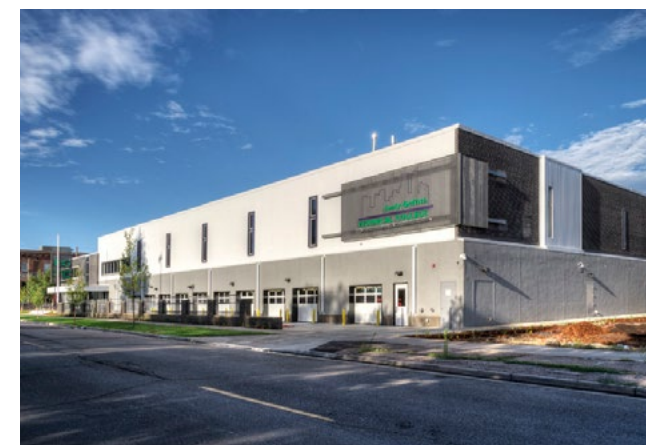
Exterior of Building
