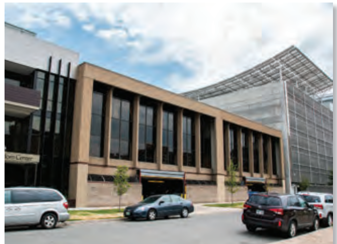
West elevation. Photo by: Milender White
