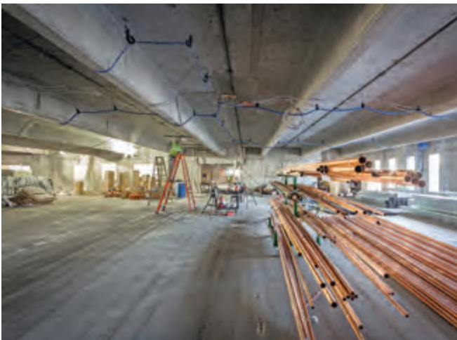
Work progresses on the third floor Photo by: Ben Eyster
