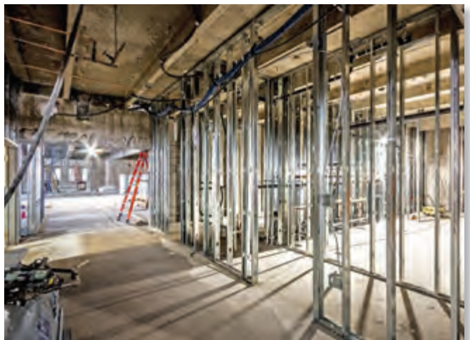
Third floor framing for offices. Photo by: Ben Eyster
